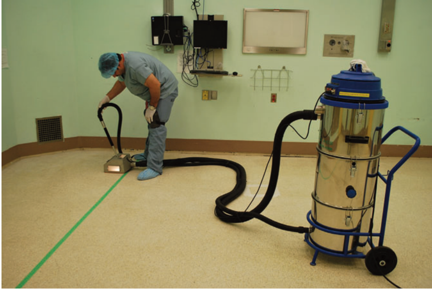
Tornado ACS works in the most sensitive environments; shown here restoring a hospital operating room floor.
