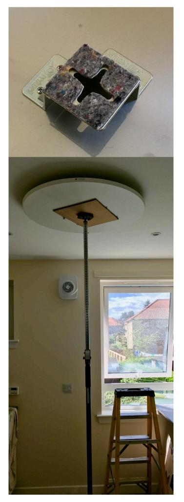
Ensure the self adhesive pads are installed to the brackets on the rear of the heating panels as indicated opposite
