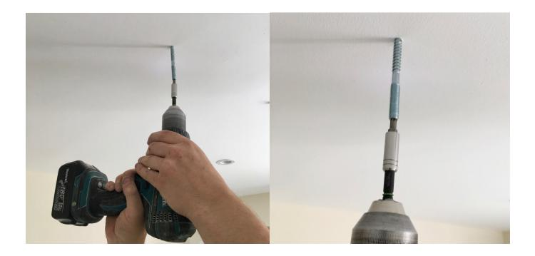
Fix dowel screws through plasterboard ceiling into suitable pre-installed timbers leaving approximately 25mm of M8 thread protruding to accept M8 Mudguard Washers and Nyloc Nuts
