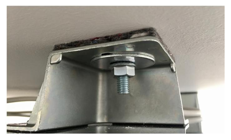
Install M8 Mudguard Washers and M8 Nyloc Nuts to each threaded dowel screw and tighten to very slightly compress the pre-installed self-adhesive pads. Once all fixings are secured remove support.
