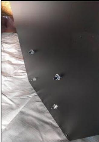
3. Set the steel plate in desired location on floor with the bolts sticking upright. (The flat head of each bolt will be recessed in the underside of the steel plate. See Figure 5.)
