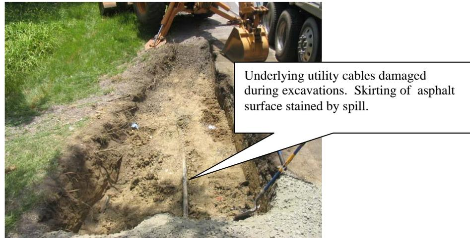
**Figure 6. Showing underlying cables and stained skirting of pavement.**
