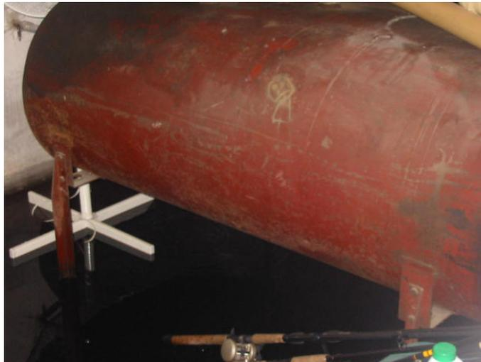
**Figure 1. Release of heating oil from the tank**
