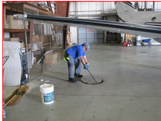
Oil water separators at airports
