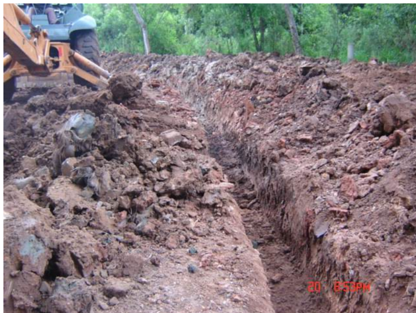
Figure 2. Construction of irrigation canals
