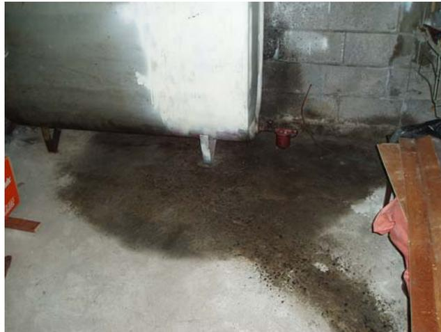
**Figure 1. Stain on concrete seen even after repeated washing**
