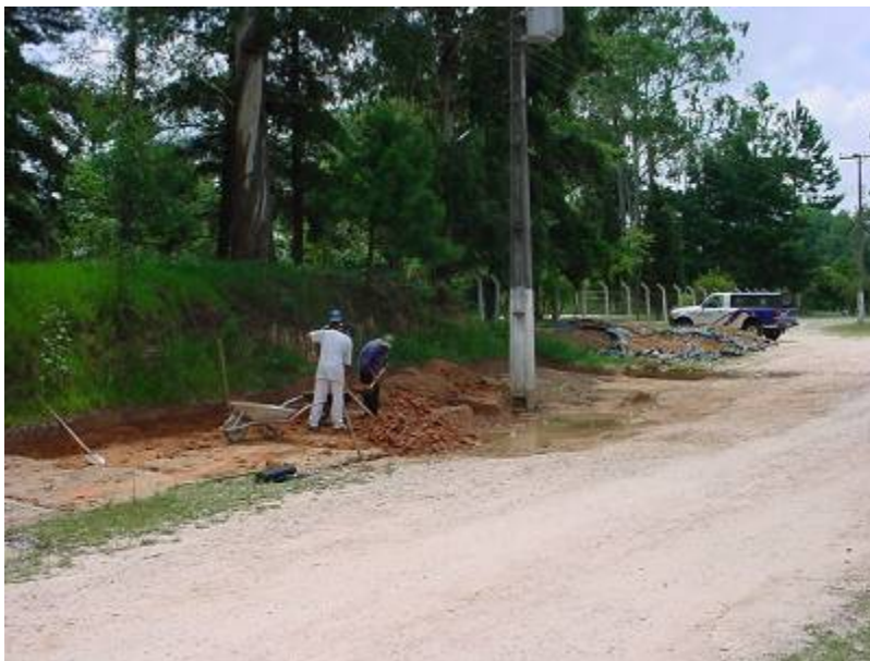
Figure 2. Excavation of the contaminated soil.
