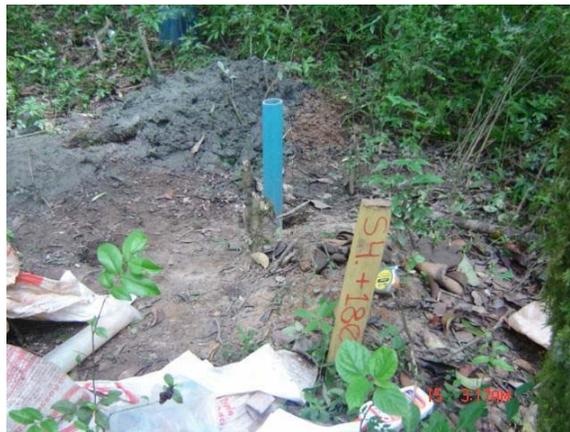
**PLATE 2. INSTALLATION OF MONITORING WELLS**
