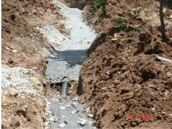
**PLATE 3. LAYING OF PIPE FOR PUMPING WATER/AGROREMEDIATION**
