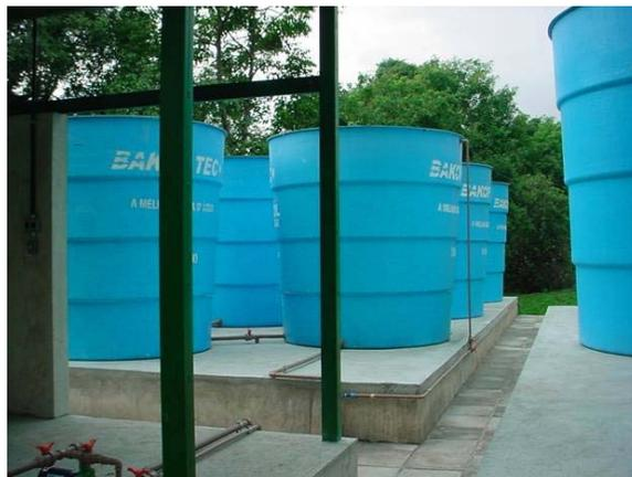
**PLATE 5. HOLDING TANKS FOR COLLECTION OF WASH WATER FOR FURTHER TREATMENT TO REDUCE TPH LEVELS TO ACCEPTED VALUES BEFORE DISCHARGE.**
