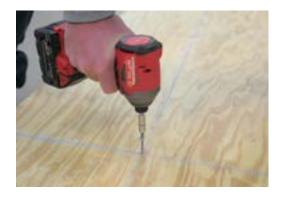
FIGURE 5: Attaching the plywood
