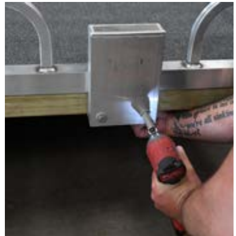
FIGURE 12: Mounting the transom
