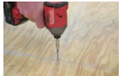
FIGURE 4: Attaching the plywood
