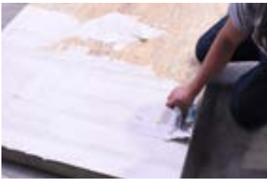
FIGURE 5: Applying the glue
