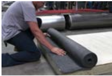
FIGURE 6: Laying the carpet
