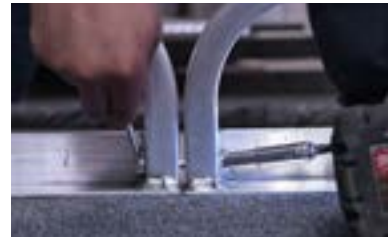
FIGURE 10: Bolting the railing
