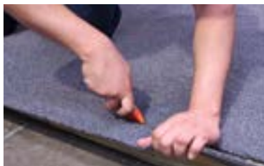
FIGURE 8: Trimming the carpet
