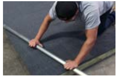
FIGURE 7: Rolling out the carpet
