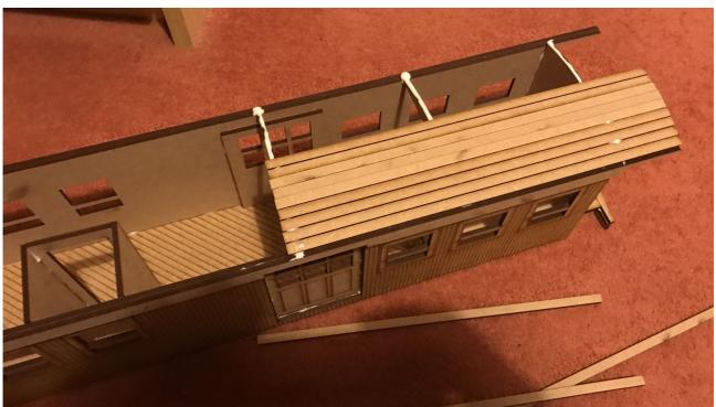
Roof time. Start with the end with the most windows. Using the roof planks as a rough guide, glue the roof supports into the model. We recommend two for this section. The roof planks are glued across the model and sit flush with the end of the model. To aid with alinging them, see the next step.
