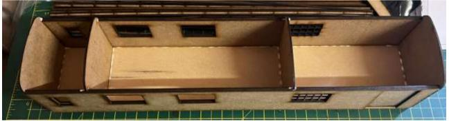
Next, glue the sides and ends onto the body. The ends have notches cut into them for the sides to slot into. Then glue into place the 2 internal partitions as shown above.
