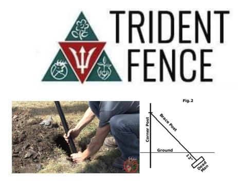
Dig a hole 1' deep where the brace post contacts the ground. Place a dead man (cinder block, large brick, or stone) in the hole perpendicular to the brace post. Wedge the brace post against the block to provide support for the vertical end post.
