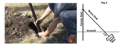
Dig a hole 1' deep where the brace post contacts the ground. Place a dead man (cinder block, large brick, or stone) in the hole perpendicular to the brace post. Wedge the brace post against the block to provide support for the vertical corner post.
