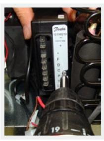
Disconnect all wires from ECU, unscrew it (one screw) and with the help of a screwdriver push the connector towards left side. Reverse the procedure to install the new ECU
