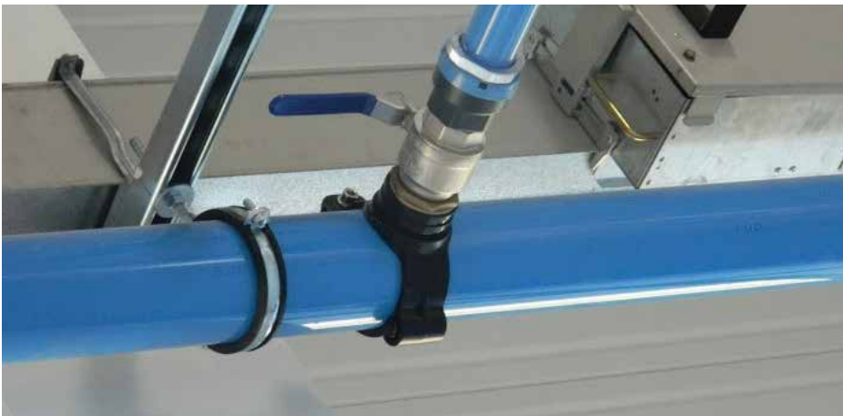
Typical Application for Saddle Branch
