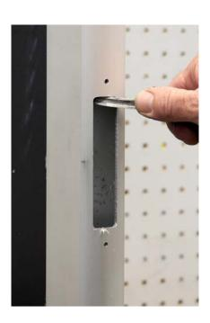
Clean the area of left over cutting lube and chips. Use a machinist scraper or an aluminum cutting file and deburr all of the openings.
