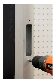
Counter sink the two mounting holes to fit the screws supplied with the flush bolt.
