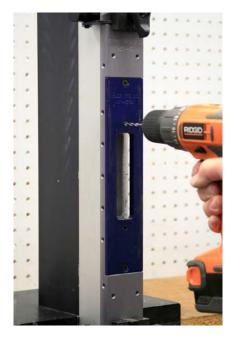
With the Clamp still attached to the door, drill the mounting holes for the flush bolt with a 5/32" drill bit.
