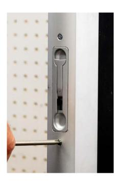
Install flush bolt into opening and secure with the factory supplied screws. Don't forget to adjust rod height prior to installing.
