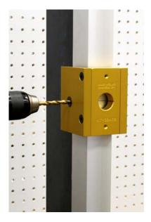
Leave the 1/4" bit in and drill the pilot hole for the outside rim cylinder. Once all holes have been drilled with the drill guide, remove from door.
