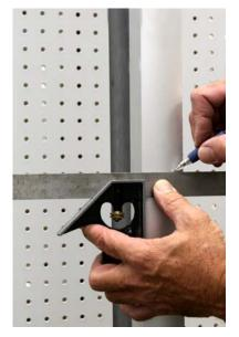
To start the installation, decide the height the panic bar is to be mounted. With a combination square draw a pencil line across the door edge at the determined height.
