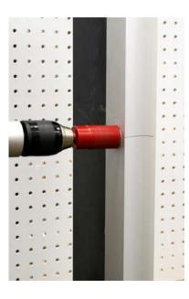
Using a 1-3/16" hole saw, redrill the outside 1/4" pilot hole. Completed hole shown on the right.
