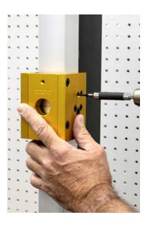
Use the drill screws that were supplied with the guide and attach one screw at the top and one at the bottom using an electric drill. Make sure the two Phillips screws on the inside of the guide make contact with the door edge and the inside plate is flat against the door.
