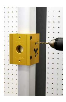
Use a 5/32" drill bit to drill top and bottom mounting holes. These holes are used to mount the panic bar with self threading screws supplied by Adams Rite.
