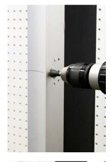
Change to a countersink and countersink the two rim cylinder screw holes per Adams Rite installation directions.
