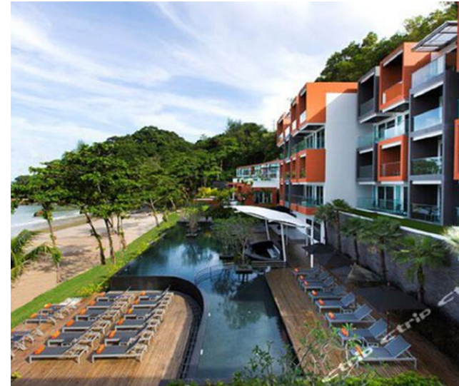
Novotel Comcala Beach, Phuket, thailand 180 rooms
