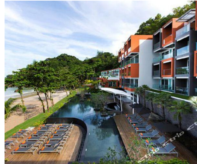
Novotel Comcala Beach, Phuket, thailand 180 rooms
