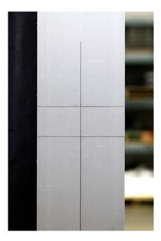
Pencil lines showing the center line of the jamb and the height of the bolt when locked have been established.
