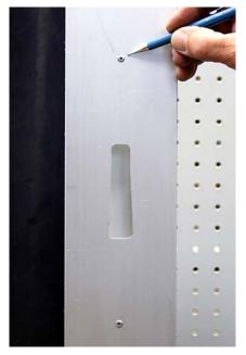
Finished installation showing mounting holes filled with a pop rivet.
