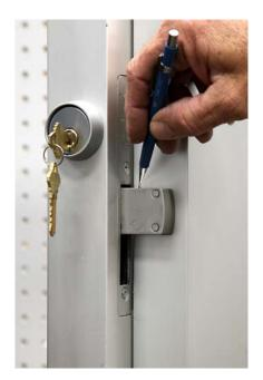
For height alignment, throw the bolt and close the door until it makes contact with the door jamb. Use a pencil and mark the top and bottom of the bolt.
