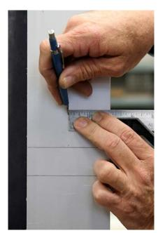
Find the center line of the jamb. This example shows the center line on a 4" wide center hung door. The center line is 2". Use a combination square and draw a vertical line at this point. Note: The center line on an offset hung door will be half the distance from the door stop to the outside of the jamb.
