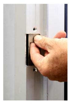
Factory mounting bracket being installed.
