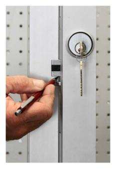
For height alignment, close the door until the latch makes contact with the door jamb. Use a pencil and mark the top and bottom of the latch.
