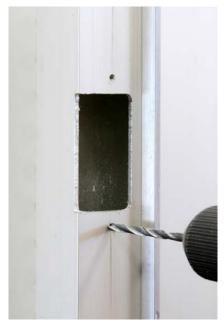
Drill out the holes left by the tek screws to 3/16". These holes will be used to mount the factory mounting bracket.
