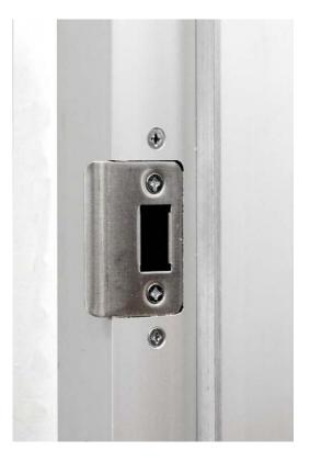
Finished installation showing strike and dust box.
