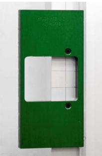
Make sure the template is square to the jamb prior to running the second screw in.
