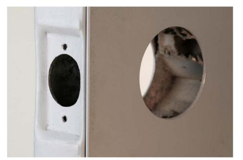
Lock prep with faceplate indention made by our Pit Bull tool. The HIT-24 will also work if you use a cut out and mounting brackets.
