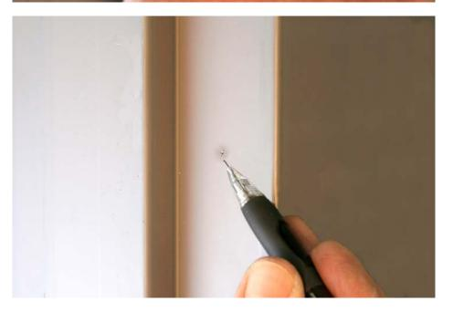
This is the exact center of the strike. Use this point to establish layout lines required for the strike cutout. See a listing of the strike mounting brackets we offer on our web site to mount strikes plates in steel jambs.
