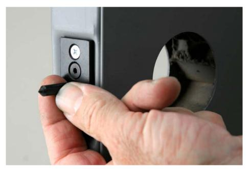
Place the locator point in the HIT-24 push all the way in and close the door.
