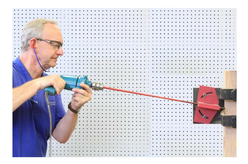
When drilling wood composition doors, use a drill speed of about 800 rpm. For best results DO NOT EXCEED THIS SPEED. Drill only to a depth of 1" to 1-1/2" then with the drill still running, pull the bit completely out to clear the hole. If drilling a mineral core door, cut the drill speed to about 400 rpm. Make sure to drill to use the same drilling methods as for the wood core door.
