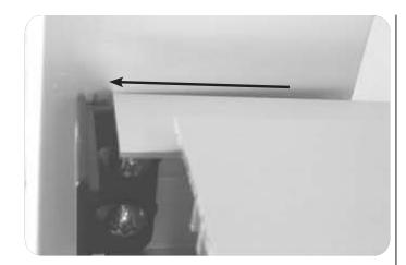
C. Attach head of device to stile with 2 ea.1/4-20x1/2 flat head screws. Tighten screws on the head and tail of the device.
