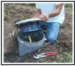
Controls mounted on plate attached to lid
