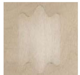
timber patching (on back face only)
