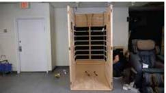
Slide the side panel and back panel together and secure with the metal latches on the outside. Slide the other side panel and secure to the back with the metal latches on the outside. Slide the other side panel and secure to the back with the metal latches on the outside.
