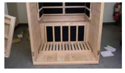
Place the leg warmer panel in the sauna with the notch at the bottom for the floor panel cable. Push the side panels in to secure the panel in place.
