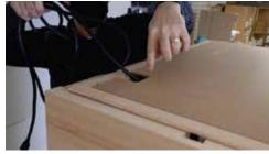
Use a step ladder to connect all the wires on the roof to the wires of the sauna, unwrap the power cord and make sure it goes through the hole in the roof cover when you re-attach it.
