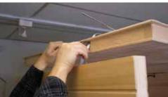
Place the roof on the sauna and ensure you thread the corresponding cables through the holes given.
