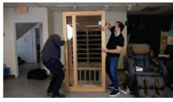
Attach the door by interlocking the latches on the side walls to the notches in the door frame. Push the door downward and it will securely lock into place.
