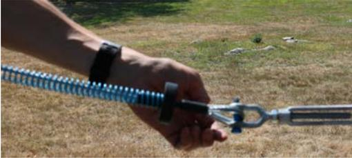
**Step 4-** Attach the other end of the zipline around the 2<sup>nd</sup> tree per the installation instructions with the U Clamps. Place the trolley on the line before you finish installation
