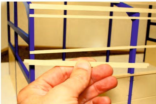
Picture Of Wall Cladding Rails:
