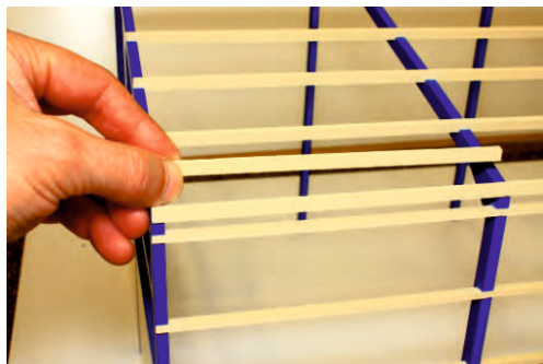
Picture of Roof Purlins:
