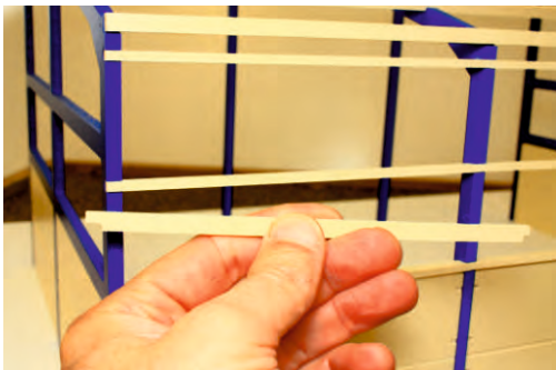
Picture Of Wall Cladding Rails:
