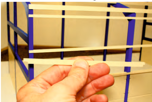
Picture Of Wall Cladding Rails:
