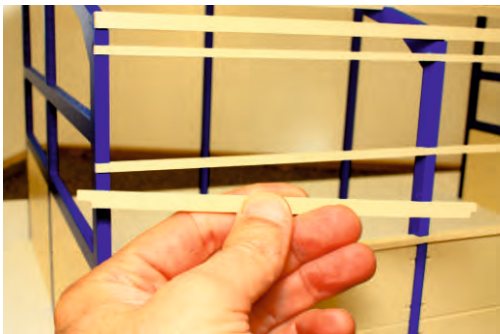
Picture Of Wall Cladding Rails:
