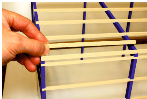
Picture of Roof Purlins:
