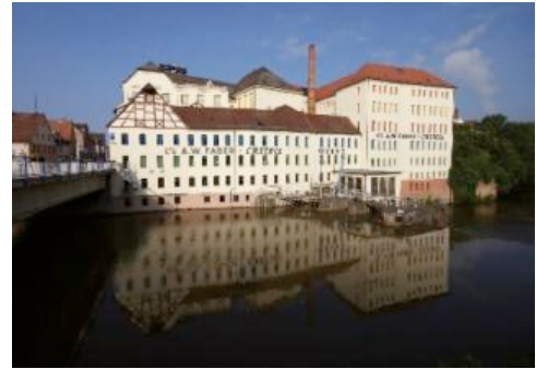
Exterior view of the pencil lead factory in Stein, hydroelectric power plant in the Rednitz river
