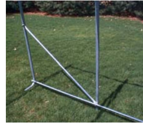
Structural wind brace on each side
