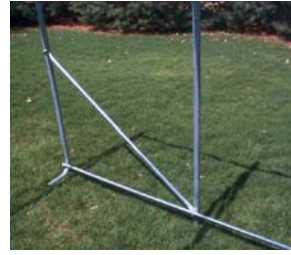
Structural wind brace on each side
