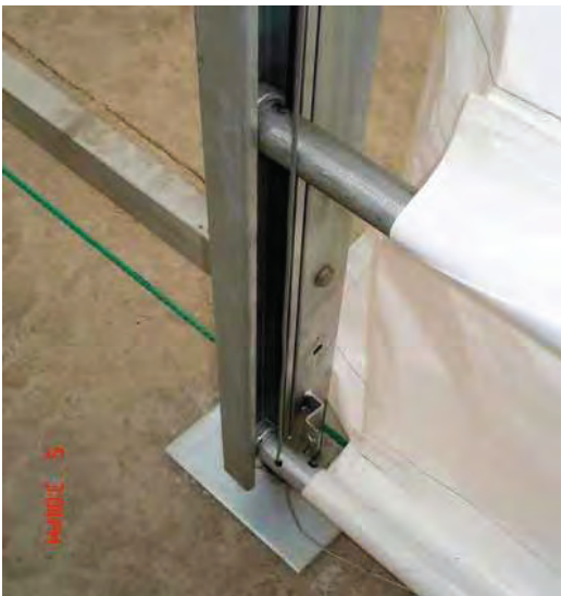
Door Tubes Inserted Into Door Track
