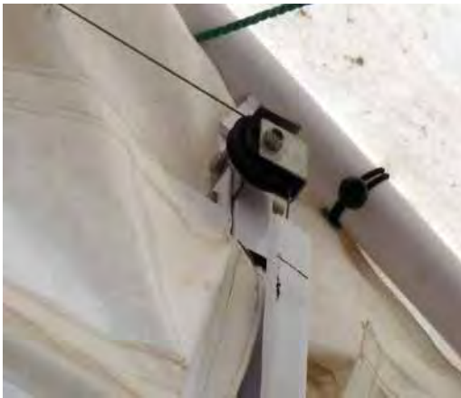
Single Door Pulley Farthest From Winch Assembly
