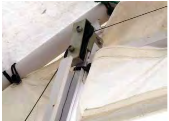
Double Pulley Nearest Winch Assembly
