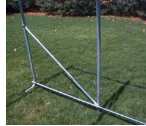
Structural wind brace on each corner
