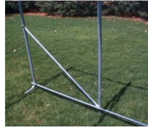
Structural wind brace on each side
