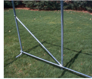
Structural wind brace on each corner
