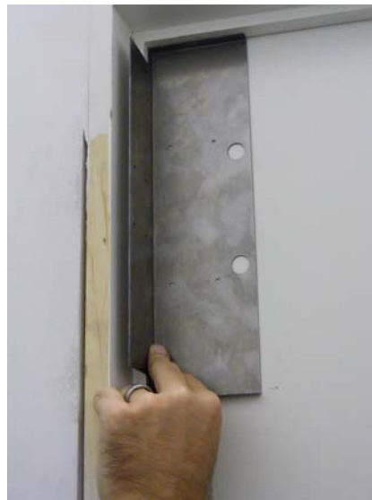
Figure 3 WR-500 lock installation template in position
