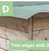
Neaten & cut excess felt
