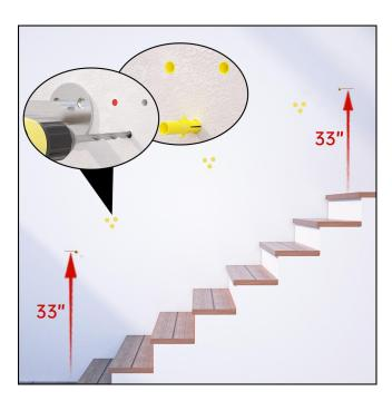
**Step 4 -** Drill guide holes with the 5/16" drill bit **3** for anchor plugs **4**.
