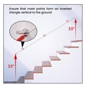
**Step 3** - Connect two thumbtacks with a piece of string, then mark the points for bracket base.
