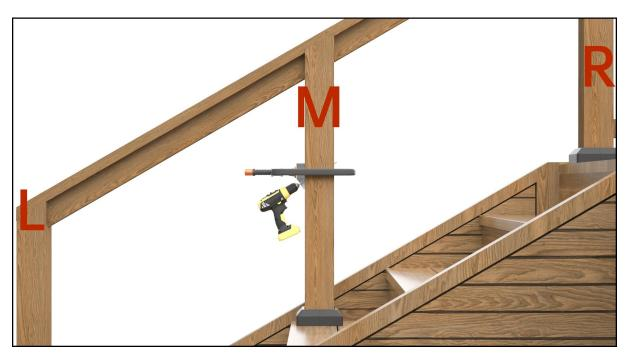
**Step 2 -** Drill 30 degrees through holes with drill guide 8 on all intermediate posts with a 9/32" drill bit.
