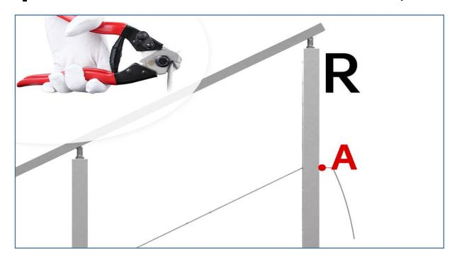
**Step 4 -** Pull the cable against the right end post, mark point A from the right side, and cut cable on point A with cable cutter 4.
