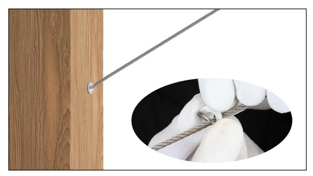
**Step 11 -** Install the adhesive washers **5** and angle protector sleeves **8**.
