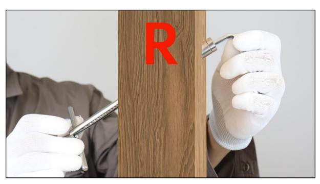
**Step 9 -** Put in angle washer **5**, tighten the tensioner **1** with an Allen wrench **1** and socket wrench **1** on the right end post.
