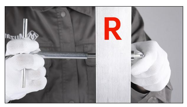
**Step 7 -** Tighten the tensioner ① with an Allen wrench ② and socket wrench ③ on the right end post.
