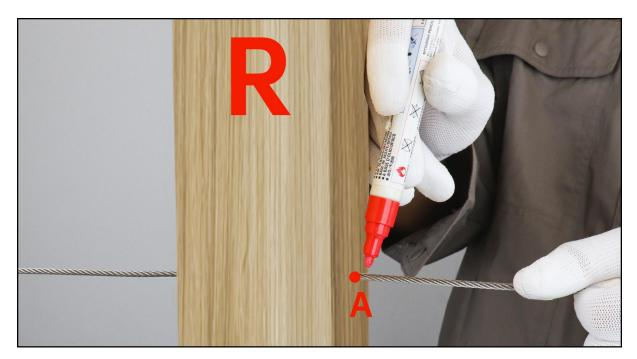
**Step 6 -** Pull the cable straight against the right end post, mark point A from the outside, and cut cable on point A with a cable cutter **3**.
