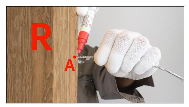
**Step 6 -** Pull the cable against the right end post, mark point A from the outside, and cut cable on point A with cable cutter **3**.
